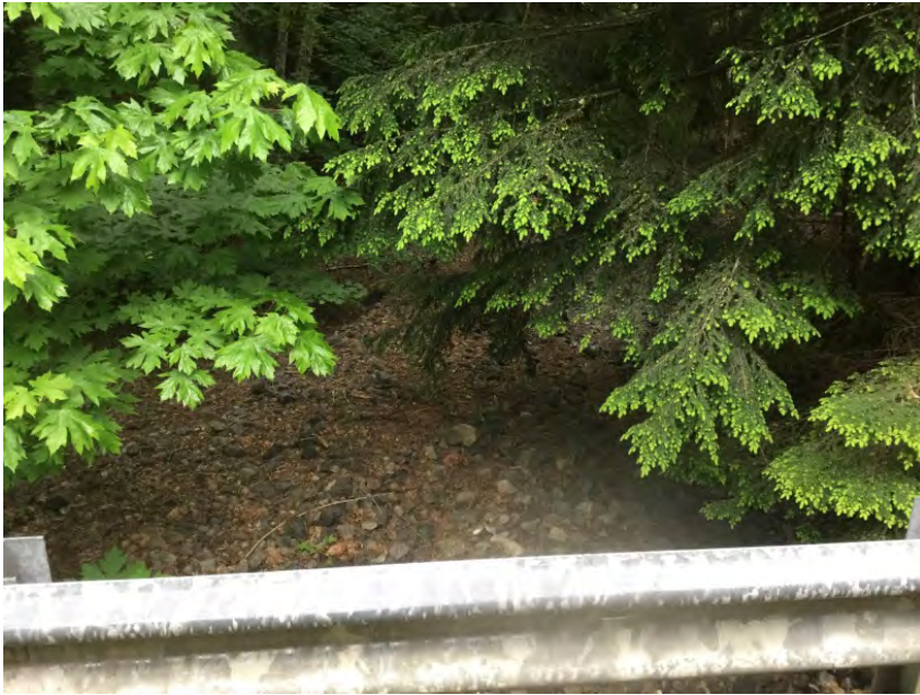
Looking downstream from deck
