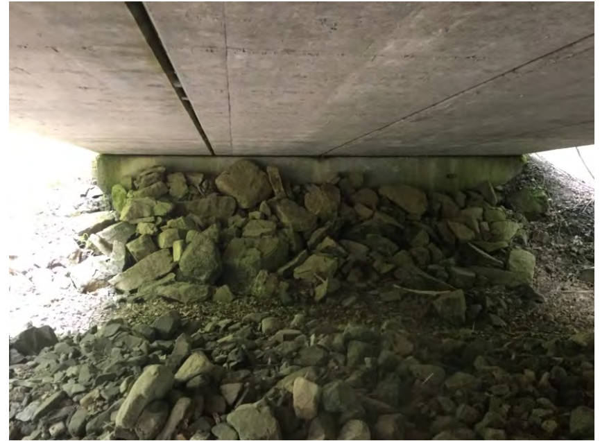
Left Bank Abutment when facing downstream
