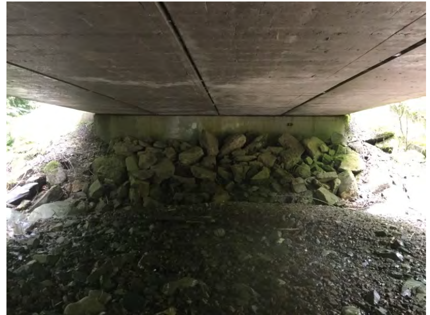
Right Bank Abutment when facing downstream
